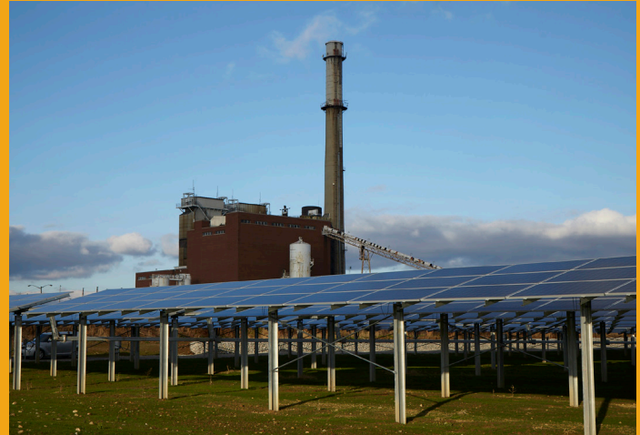
IMPA's Whitewater Valley Station and solar park in Richmond, Indiana
